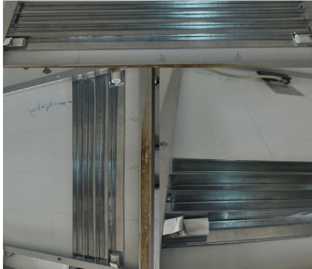
Figure III.11 Corner Installation
