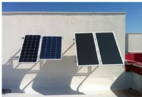
Figure I.8 Installation of monocrystalline, polycrystalline film solar panels in the hybrid energy generation system[12]
