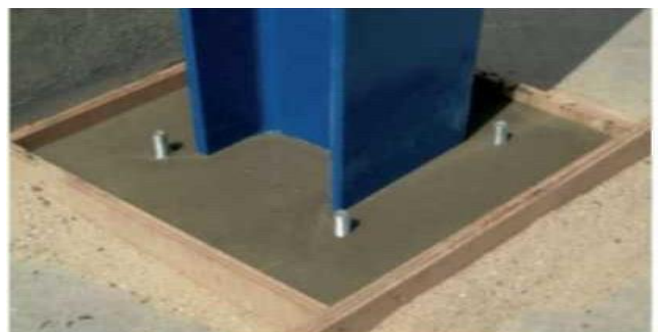
Figure I-5: Sealing and wedging [6]
