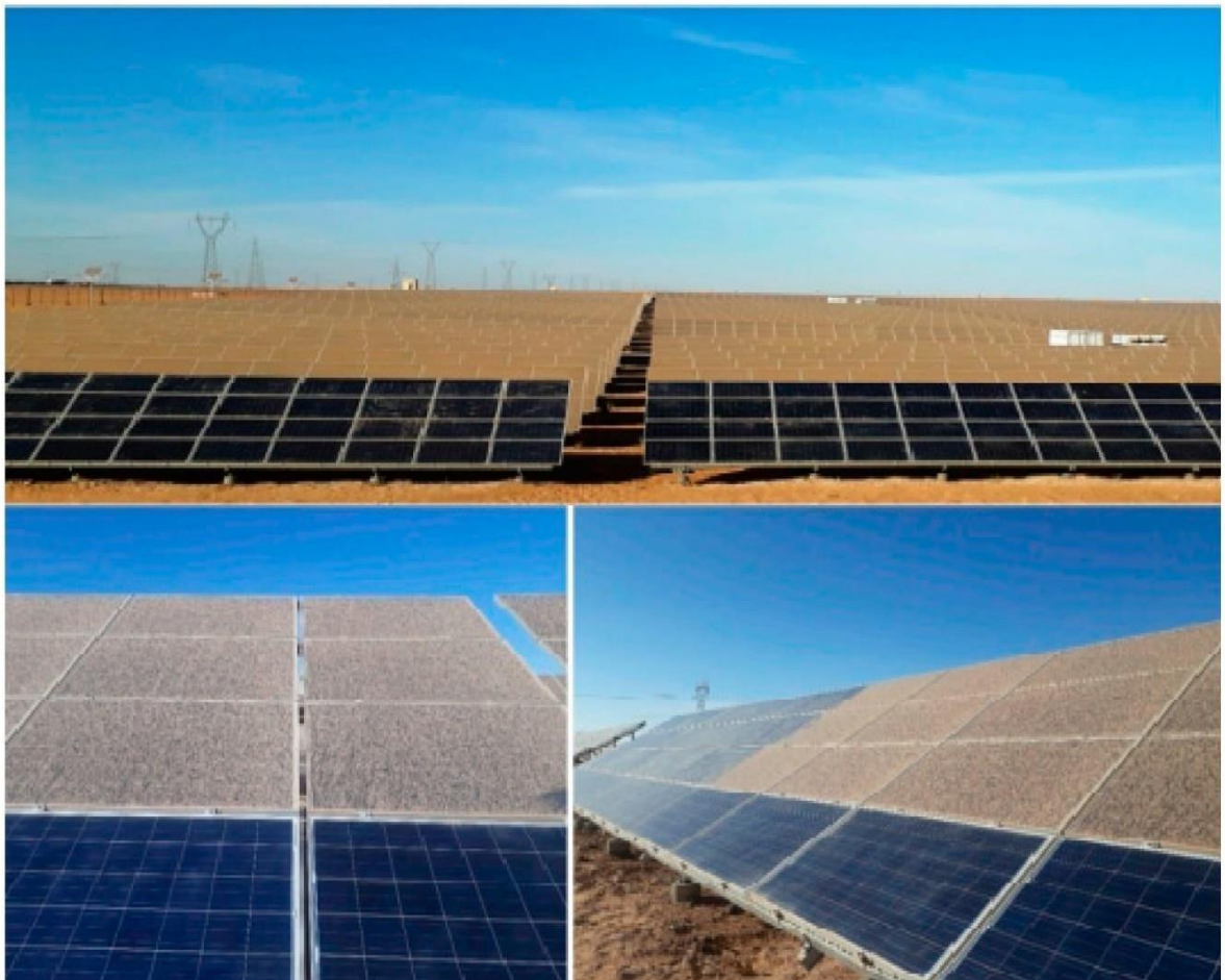
Figure 2-1 Effect of dust deposition on photovoltaic panels:
