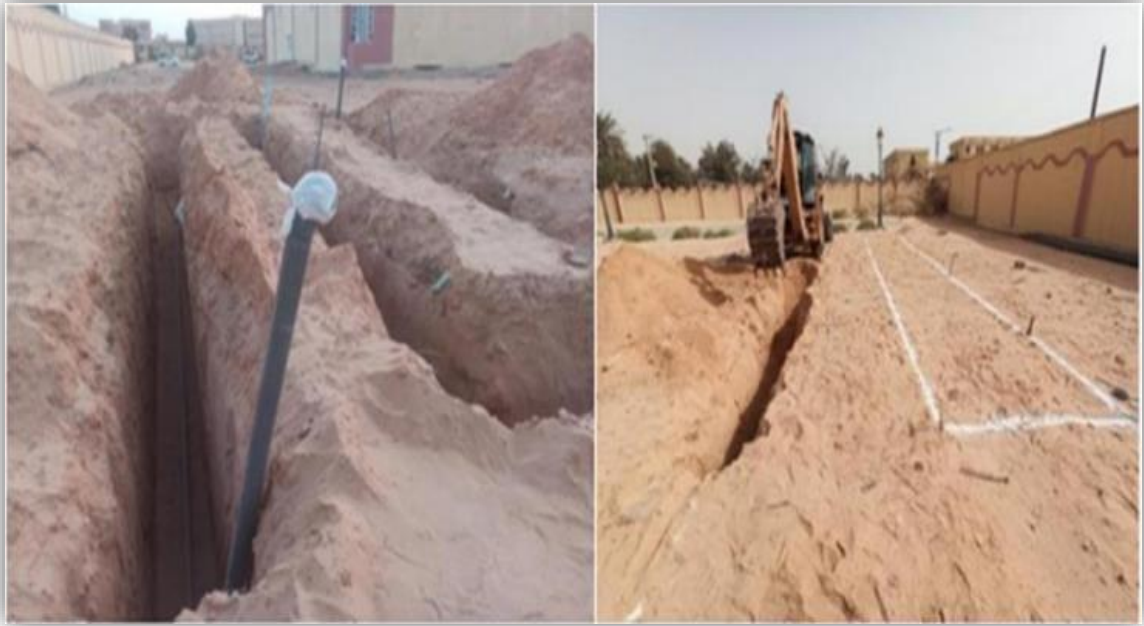
Figure 3-2: Air distribution pipes
