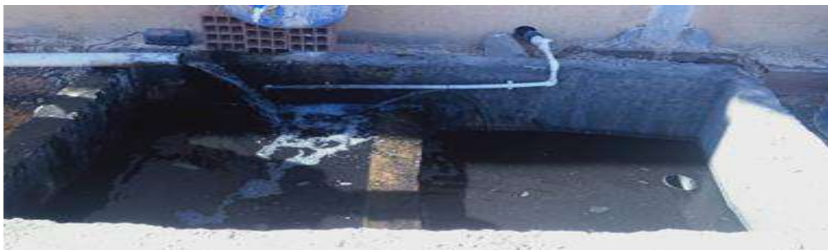
Figure III.2: Sampling Basin for Incinerator Flue Gas Washing Water – TRANSCO.
