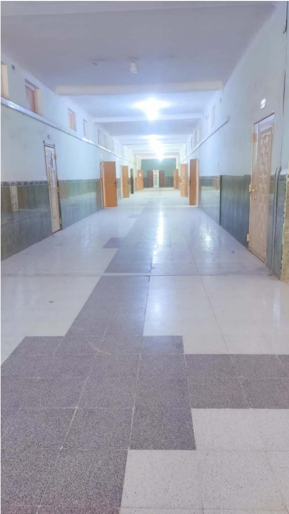
Figure 3.6: the FNTIC Electronic and Telecomm Department classroom corridor.
