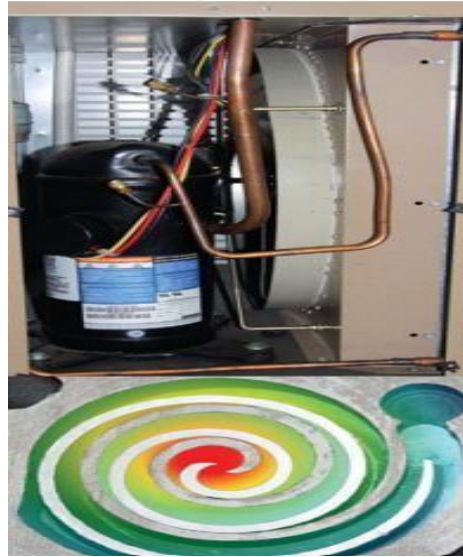
Figure I.8. The compressor raises the gas pressure and temperature by squeezing the gas to a smaller volume.
