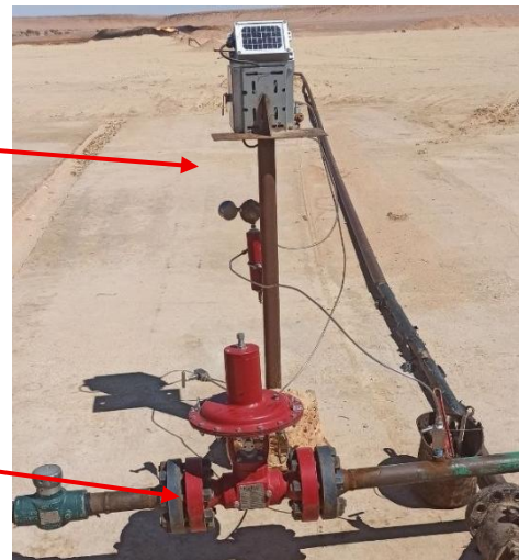
Figure II.9: Surface Intermittent Gas Lift (IGL) Injection Control System
