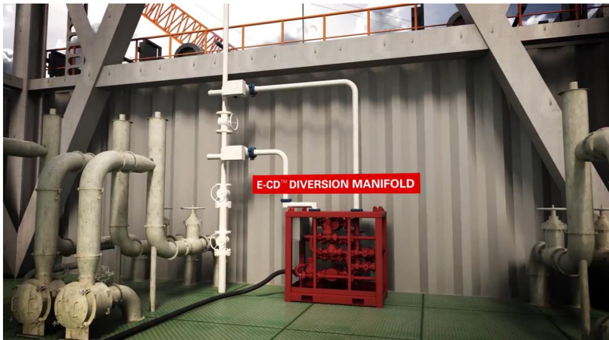
Fig.II. 6: The connection of the E-CD manifold with rig components [37].
