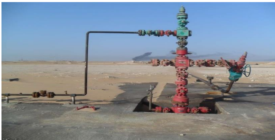
Figure 10: Complétion Gas-lift indirect
