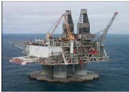
Installation marine (offshore)
