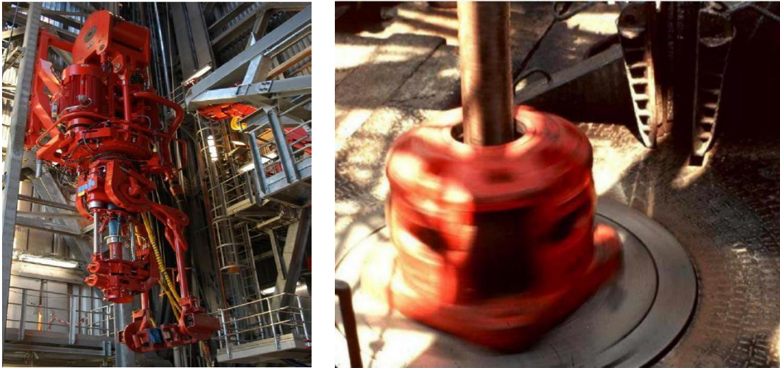
Figure I-4 Equipements de forage
