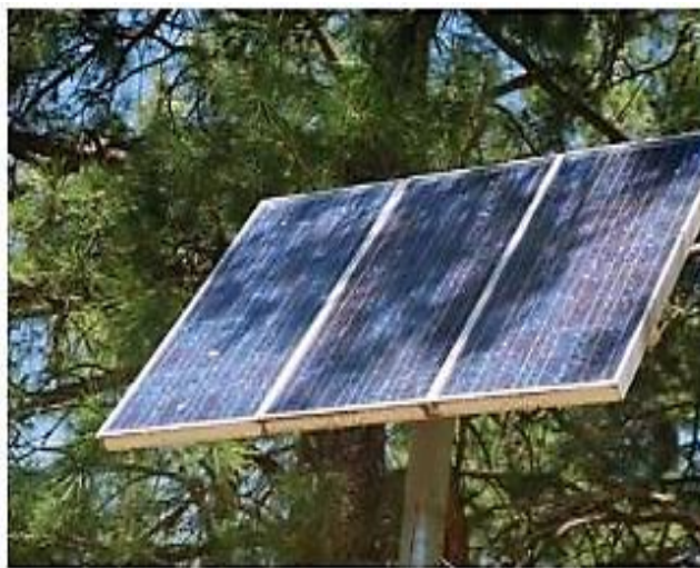
Fig I.9: PV Panel partially shaded [24].
