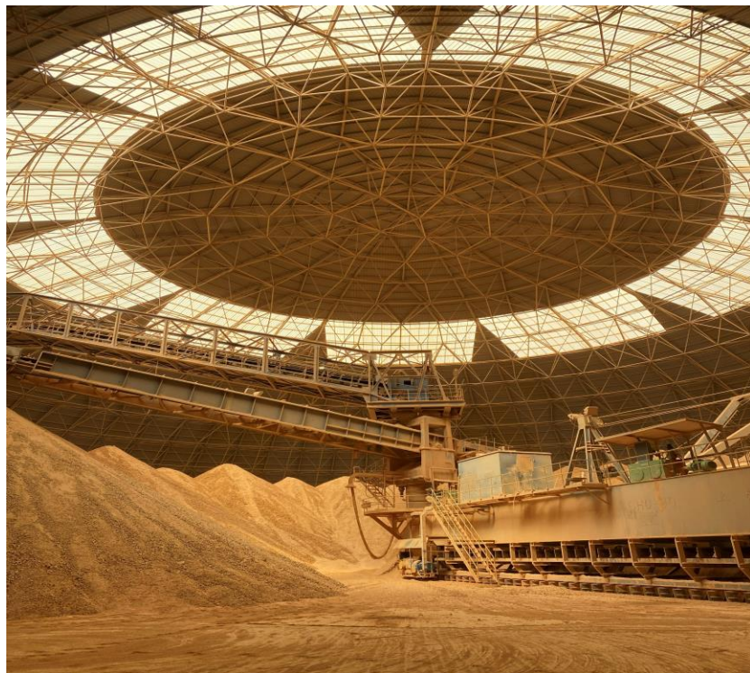
Figure 1-7 Storage of mixed materials in storage warehouses before entering the reaction stage at GICA cement plant
