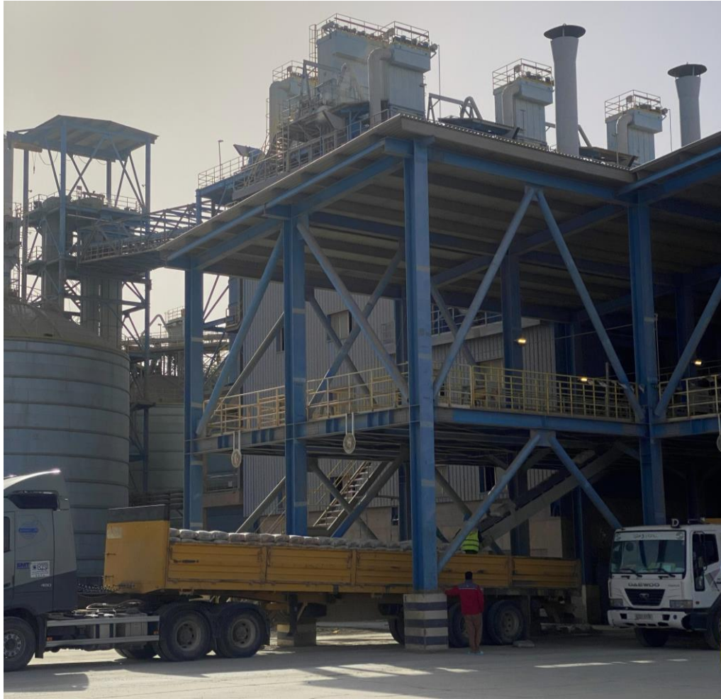
Figure 1-11 Cement factory shipping area
