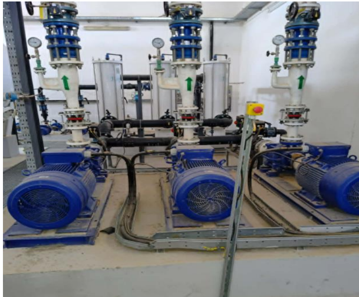
Figure II.17 : Pompe haute pression.
