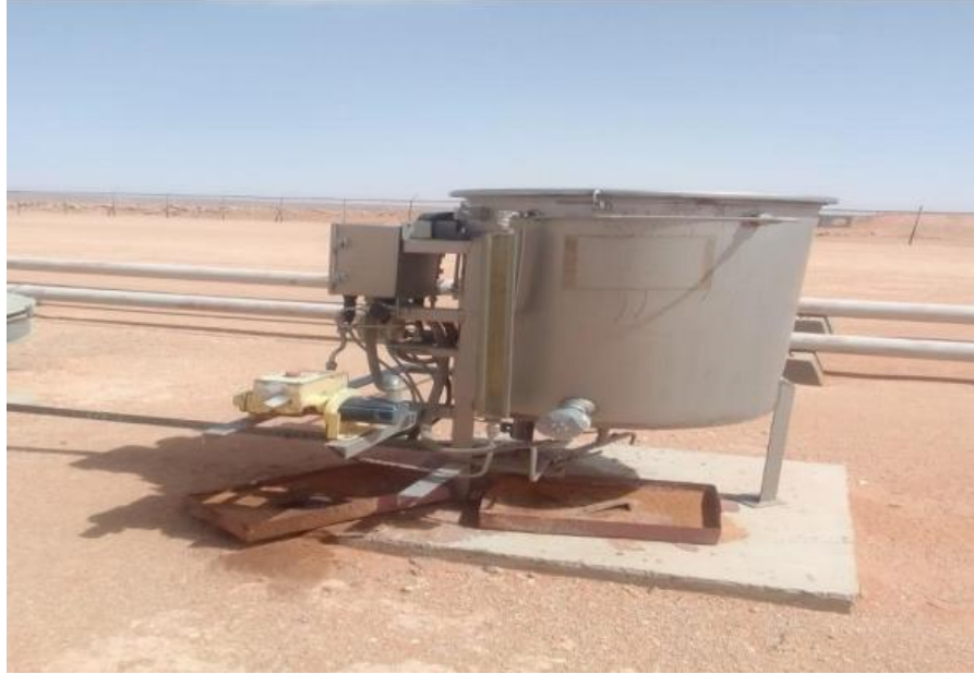
Figure III-4 : ALPHA 175INT injection Device
