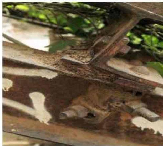
Figure I-8: Crevice Corrosion
