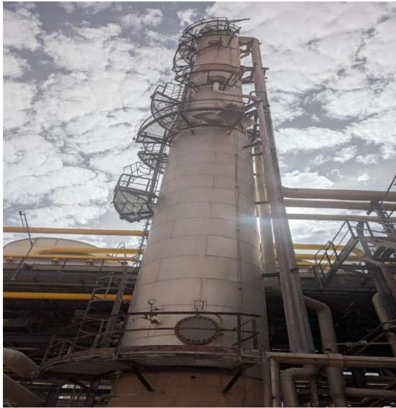
Figure.I.7. Colonne de distillation
