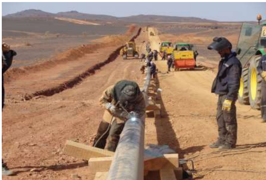
Figure 10:Field Operations and Infrastructure Deployment for the Pipeline Activity
